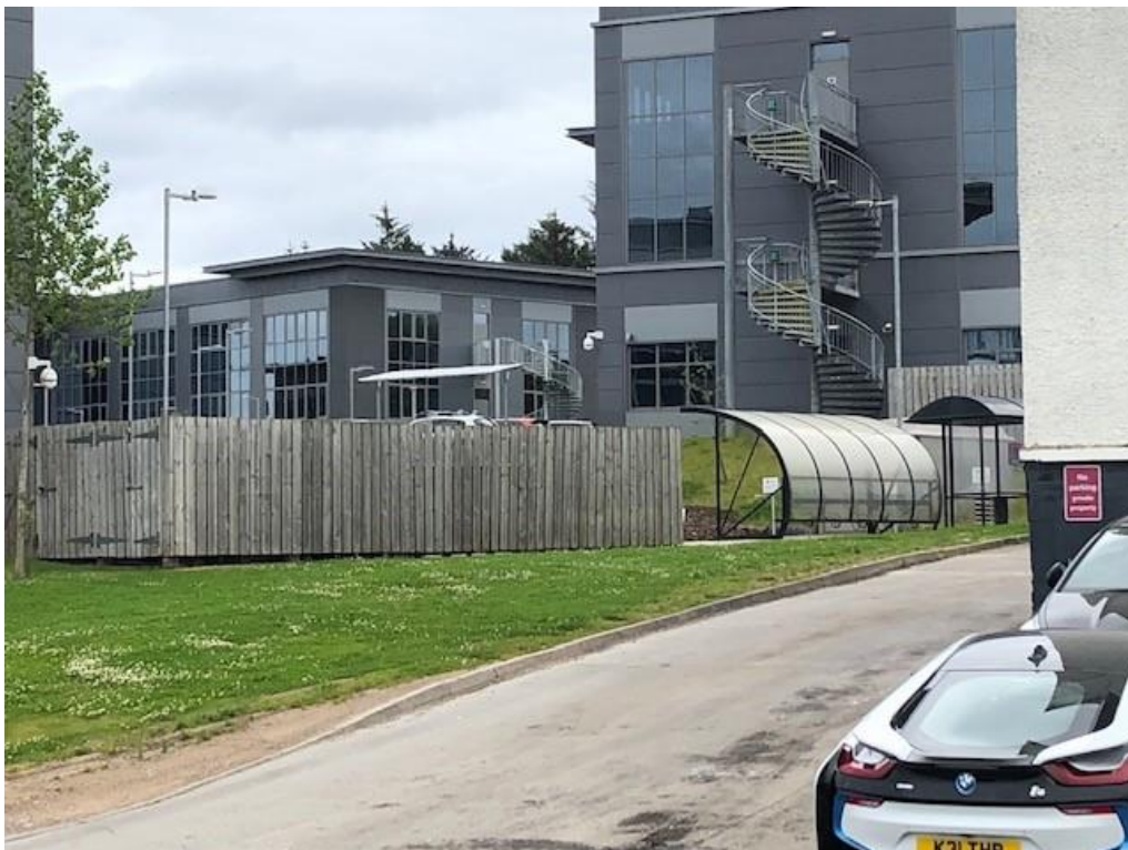
Unofficial pedestrian access.
