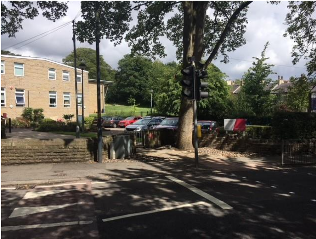
Third (pedestrian) access.
